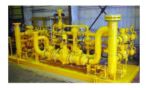
Gas Skid & Metering Module We design, install and service pressure reducing gas skid and metering modules.
