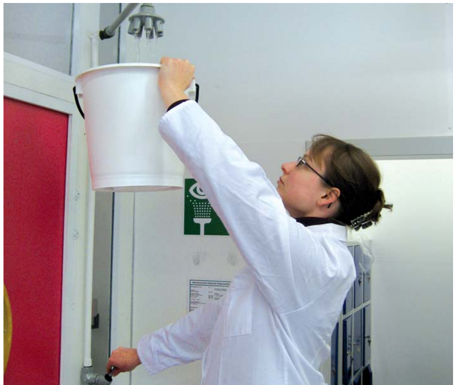
Labour-intensive water changing at every terminal point. Nowadays normal, but ineffective and expensive solutions are used to ensure the proper use as intended in buildings.
