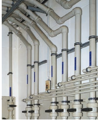
Chemical Drainage and Waste Water Treatment in PROGEF Standard, PVC-U, PEq
