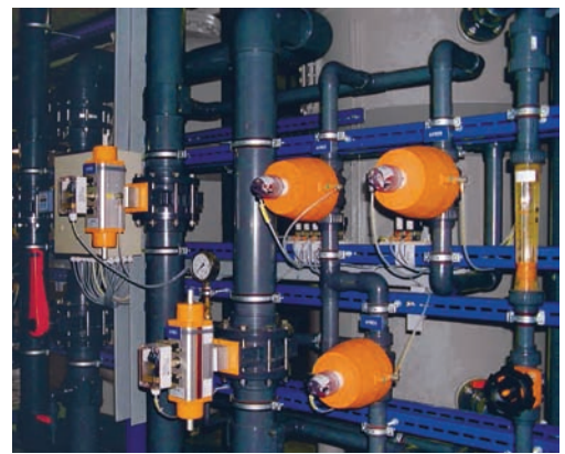
Process Cooling in PROGEF Standard, PE, PVC-U, COOL-FIT
