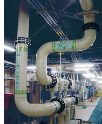
Process Cooling in PROGEF Standard, PE, PVC-U, COOL-FIT
